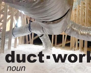
Definition: A system of metal or flexible piping containing ducts that distribute airflow From your cooling or heating system throughout you home.
